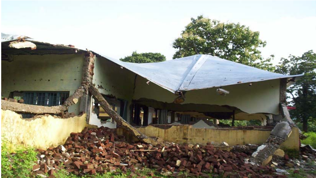
Picture 2: The roof of the Gonderas school left without support to stand
