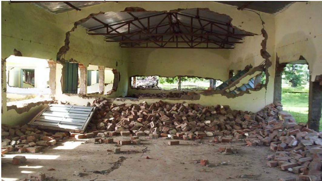
Picture 1: The demolished walls of classrooms at the Gonderas School
